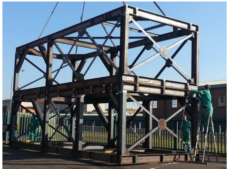
Plant structural component assembly off site at PJ Tech Middelburg
