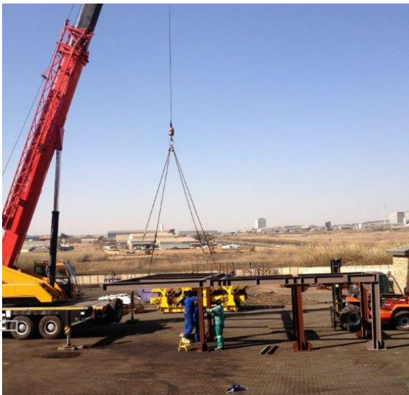
Plant component erection underway in Middelburg
