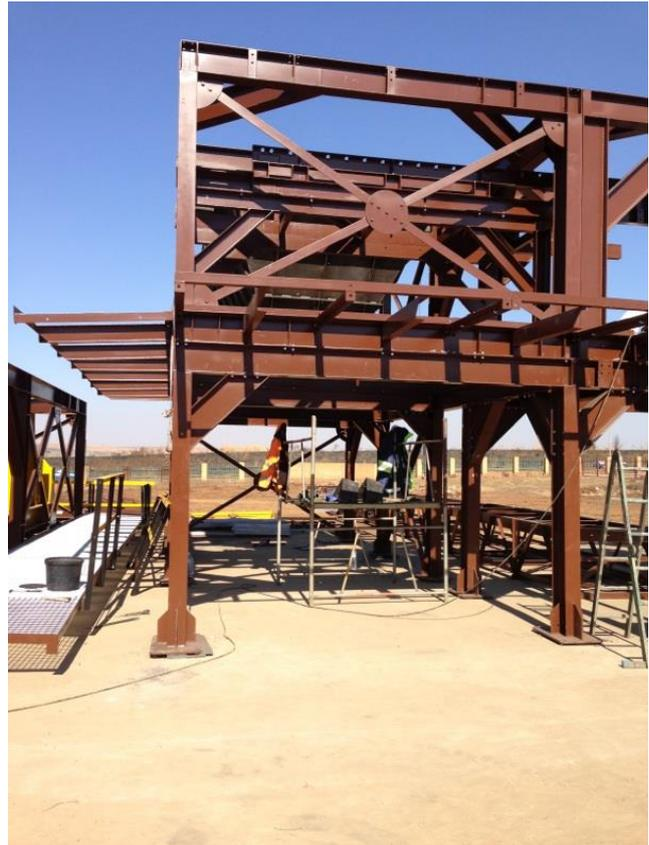
Plant structural component assembly off site at PJ Tech Middelburg
