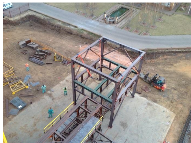
BC1/BC2 Primary crusher component assembly off site at PJ Tech Middelburg
