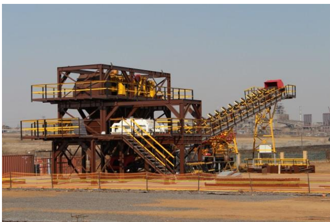
BC1/BC2 secondary crusher section erection underway in Middelburg
