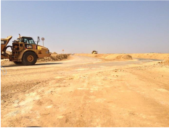
On Site pit haul roads complete with overburden stockpiling continueing
