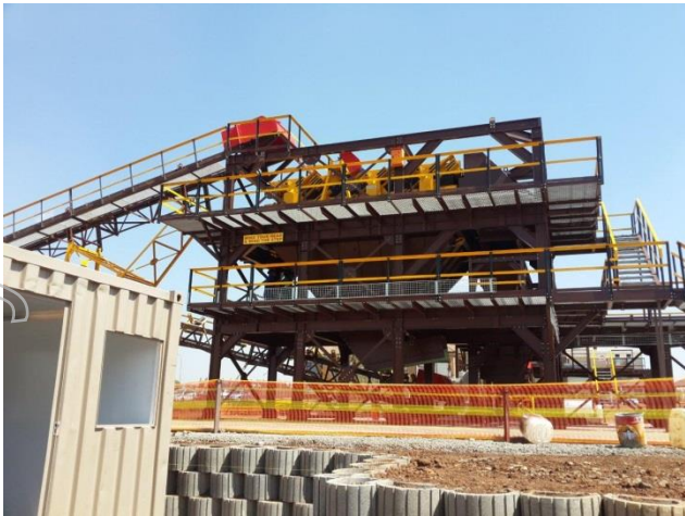
BC1/BC2 secondary crushing and screening module ready for shipment
