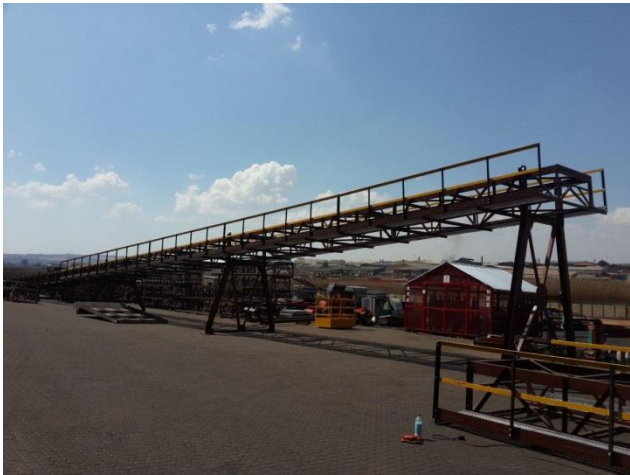
Plant conveyor component erection underway in Middelburg
