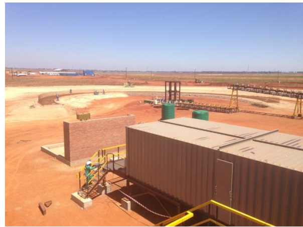
Construction of the product stockpile base
