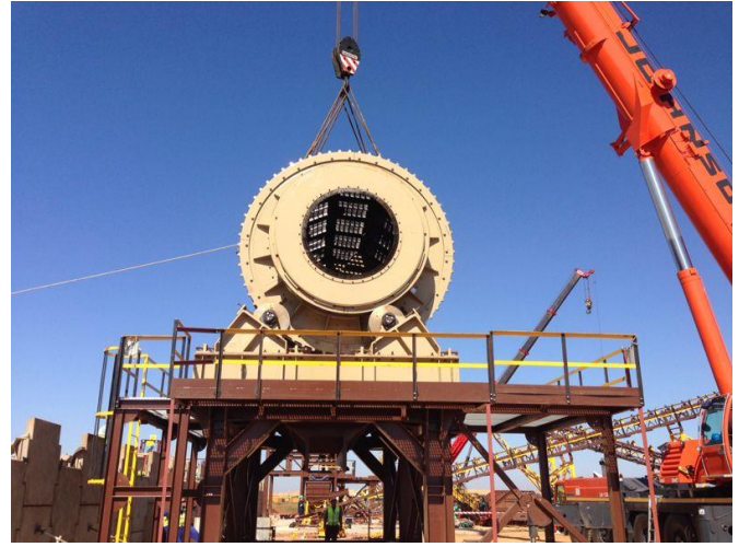
Rotary breaker installation
