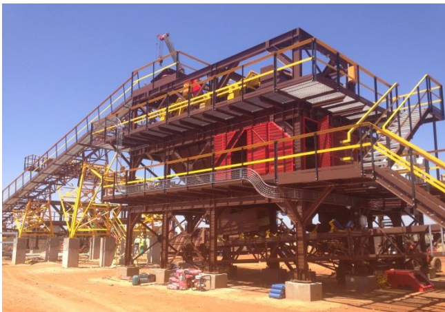
BC1/BC2 secondary crushing and screening module constructed on site
