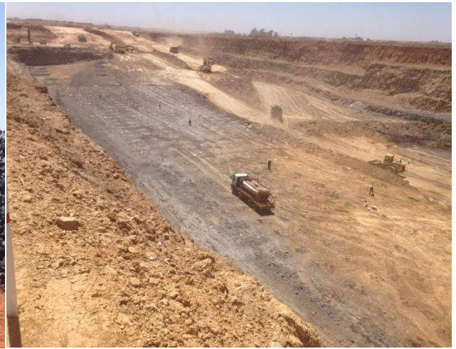
Charging of blastholes in the box-cut
