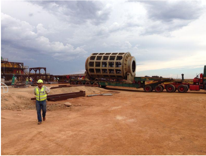
Rotary breaker arrives on site
