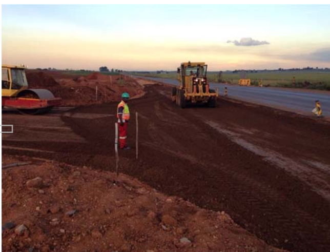
Construction of the R42 intersection
