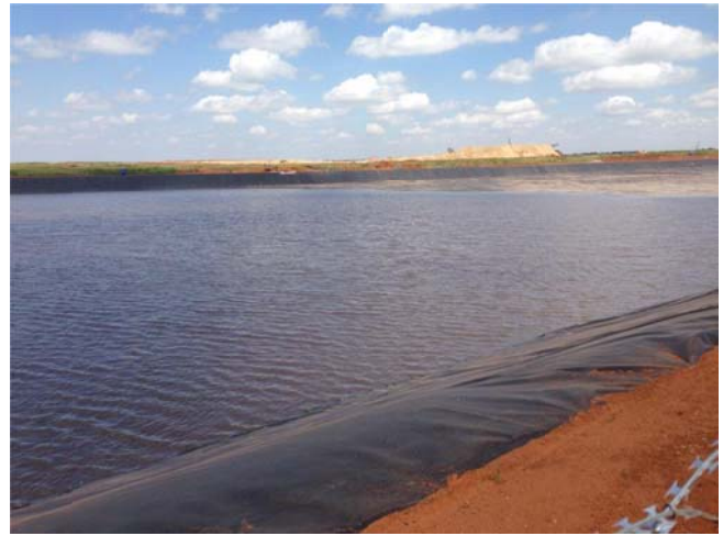
Pollution Control Dam
