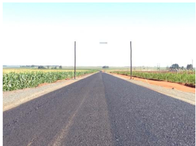
Construction of the black top surface has begun
