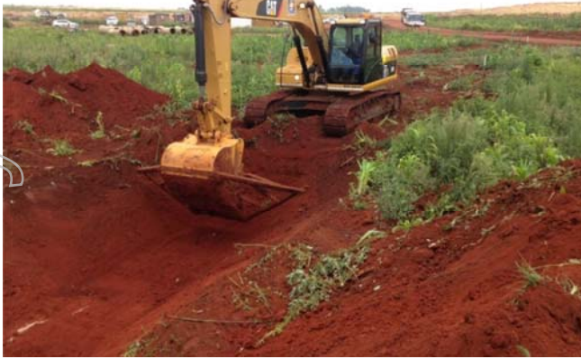
Construction of dirty water cut-off drains
