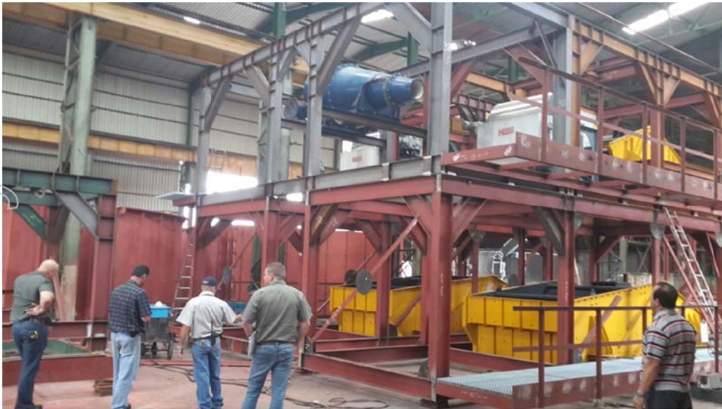
Off site construction of DMS plant continues
