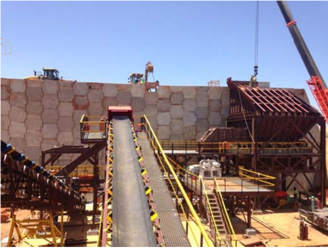
Final construction of the wing-wall at the plant
