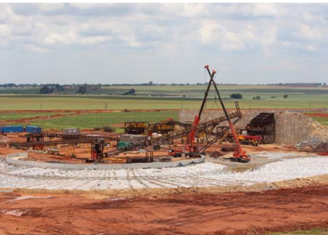
Kangala plant construction
