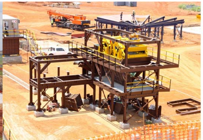
DMS plant under construction
