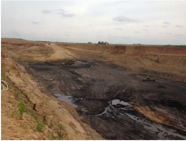
Box-cut progressing according to schedule
