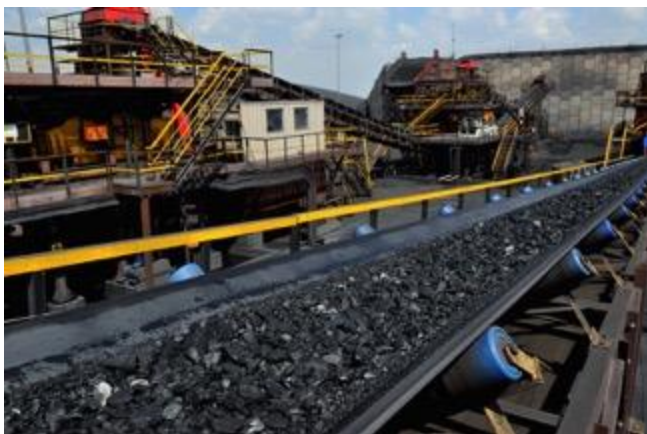
CHPP at Kangala Colliery
