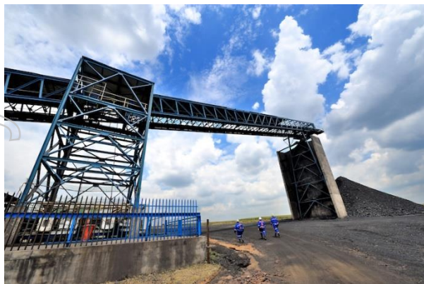
the Diepspruit shaft
